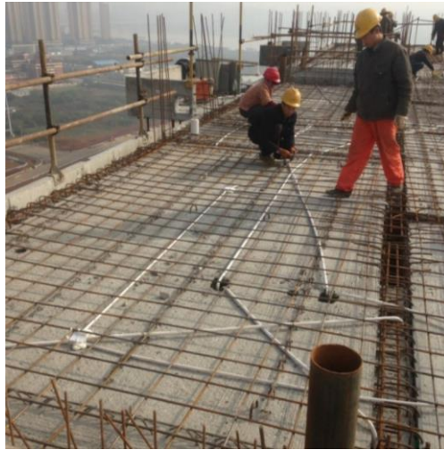
Figure 2 the video recording of the steel bar workers on construction site
